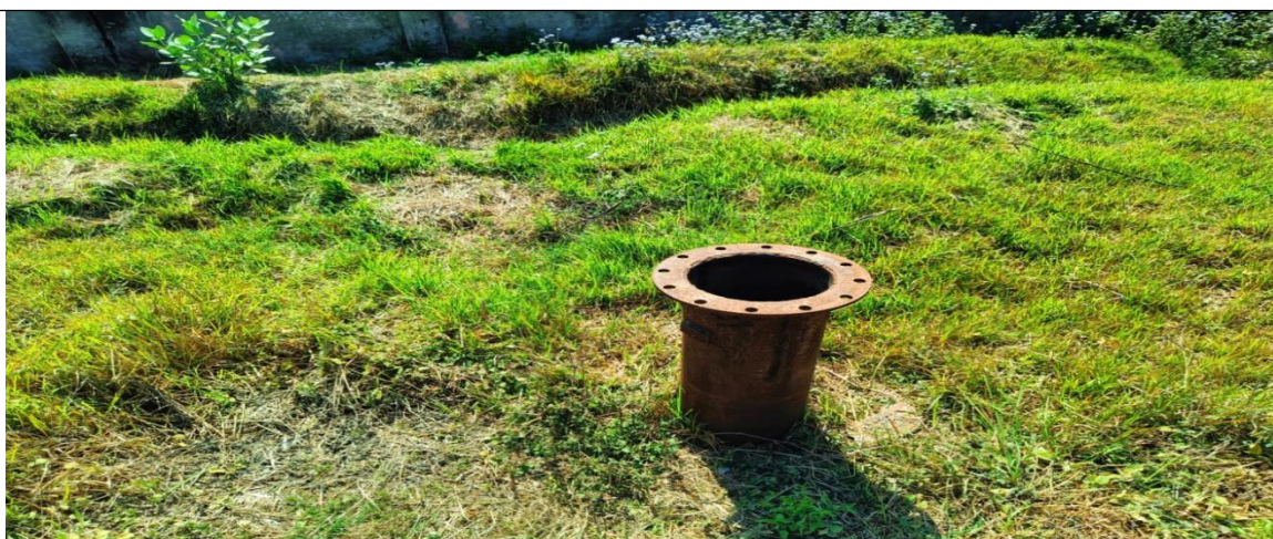
5. Existing tube well
