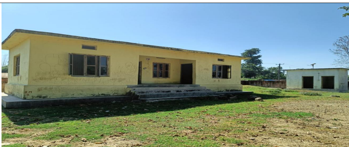
Three room Office building
