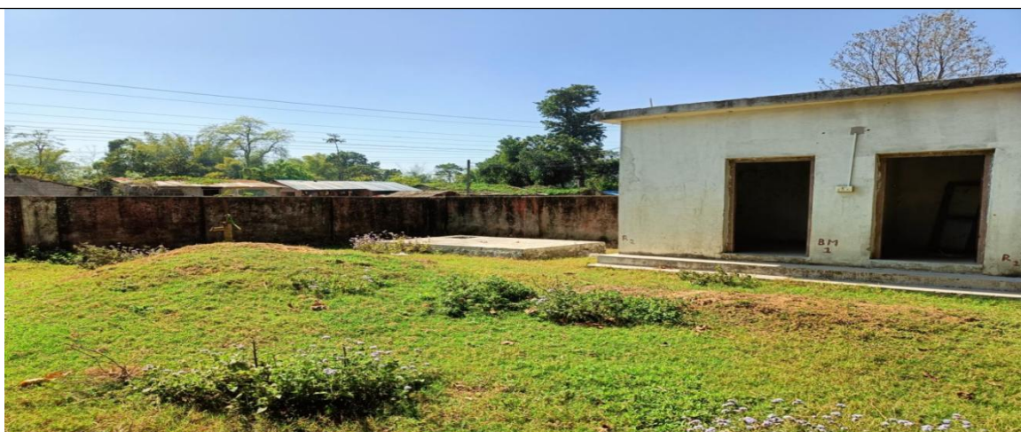
Toilet with Handpump
