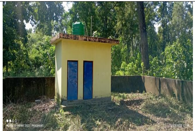
4. Toliet block with septic tank
