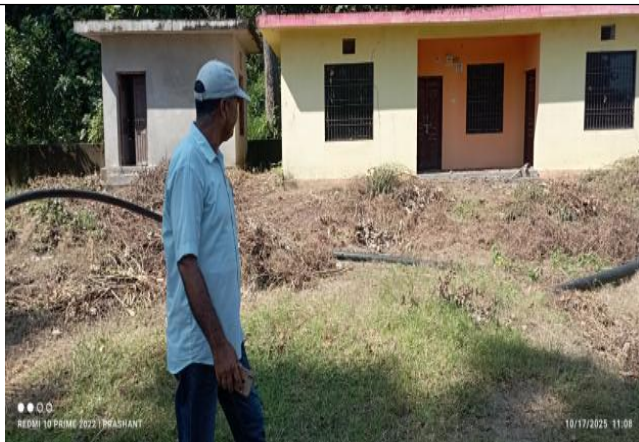
3. Three Room office building
