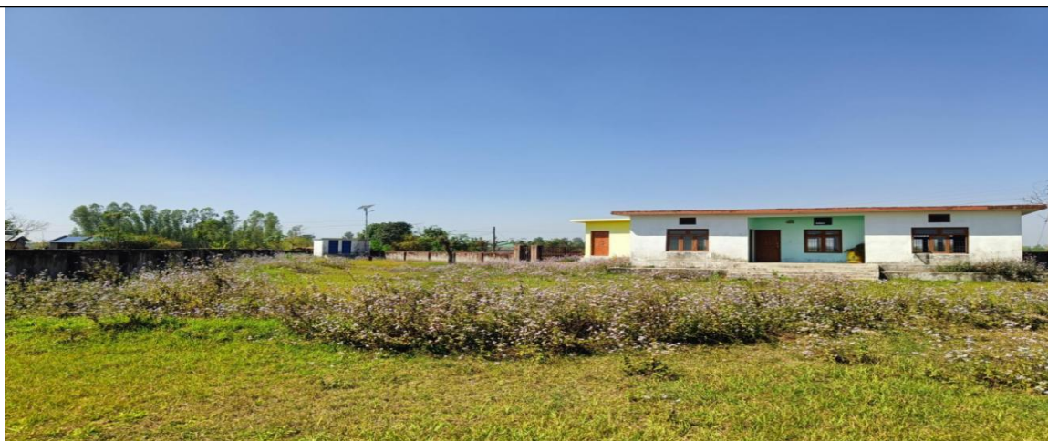
4. Existing 3 room office building of WSUC
