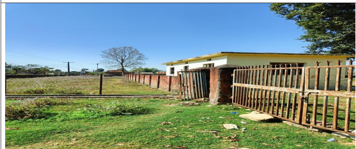
Boundary wall and Gate
