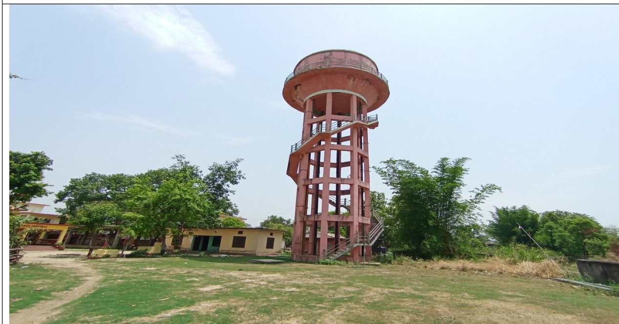
Existing structures of Durgauli WSS sub-project, OHT premises
