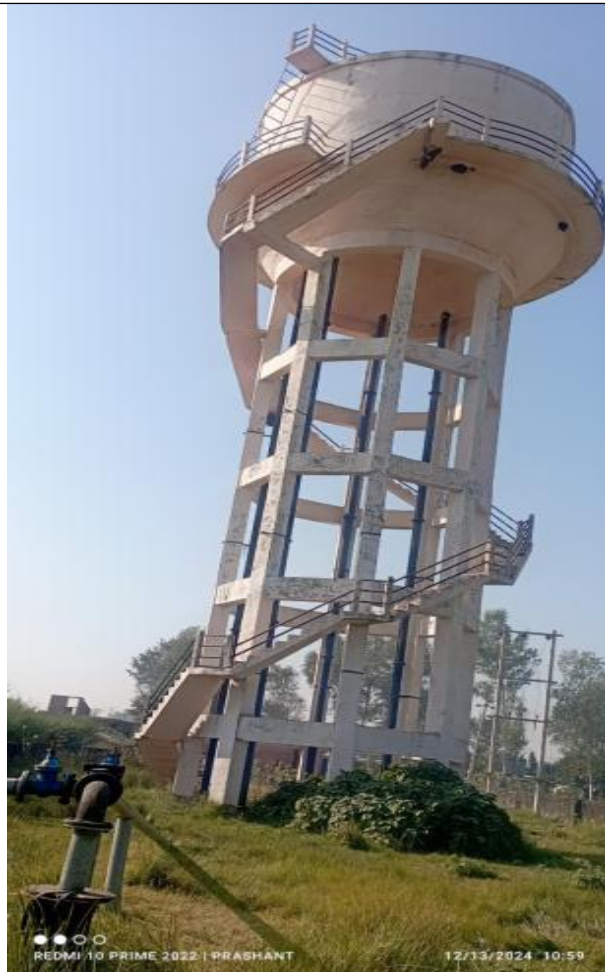
7. 1 st deep Boring at North of OHT with Transfer of 50 kVA at background
