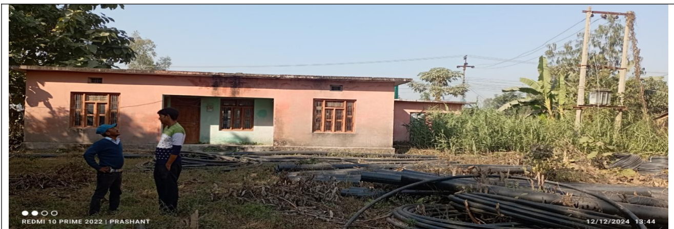
6. Existing three Room office building with 50 kVA Transformer
