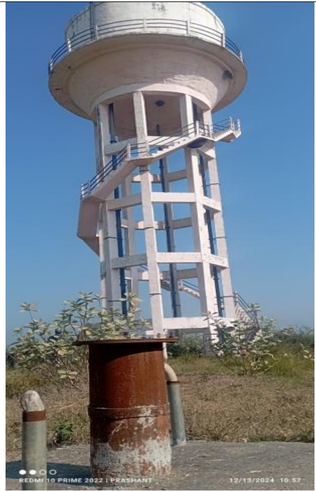
8. 2 nd deep boring at south of OHT
