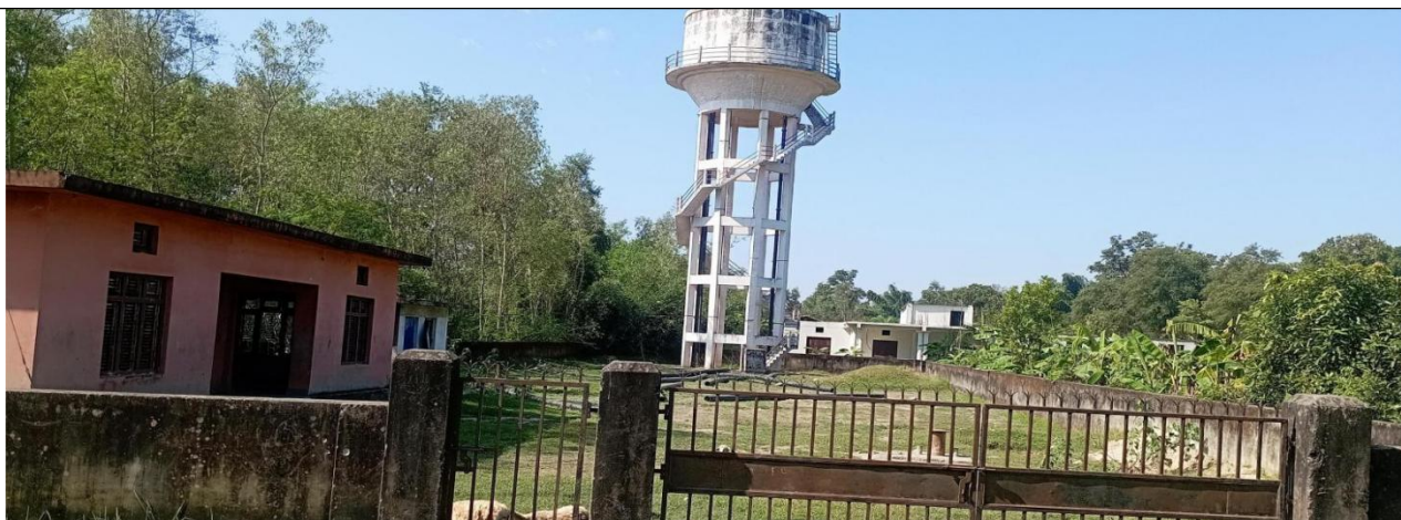
4. Existing OHT, Office building and toilet
