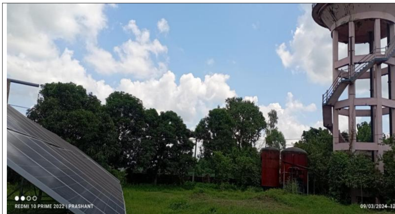
3. Existing OHT of Munuwa WSP with Solar Panel
