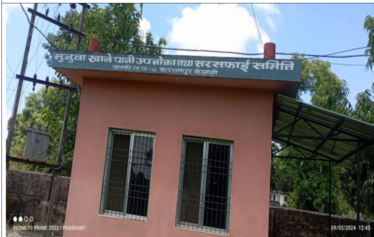
6. One room office building of Munuwa WSP with 50 kVA transformer
